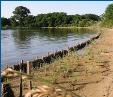
Marsh planting at grade, fiber logs near mean low water elevation
