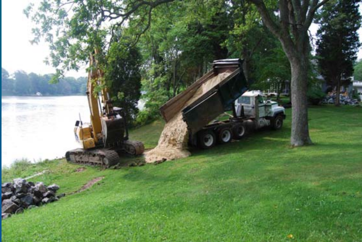
Access “ramp” for heavy equipment to haul in sand and stone
